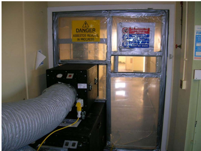
Figure 12.2 Negative pressure units and air discharge ducts, viewing panels and warning signs.
