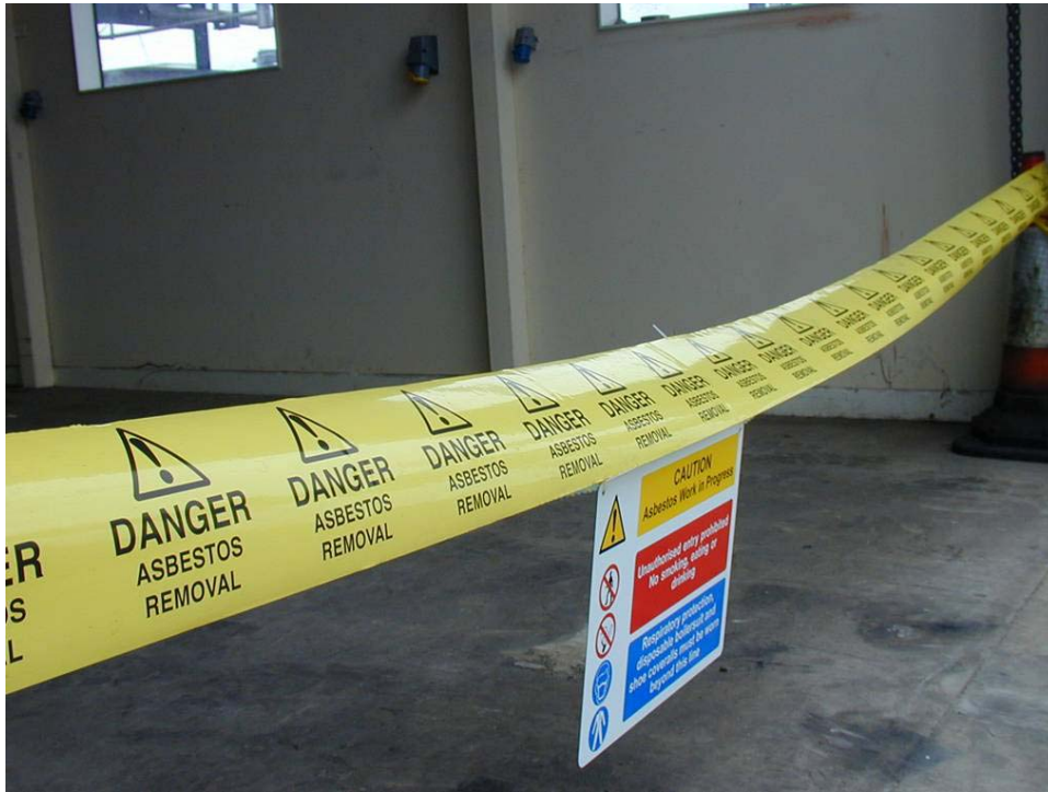
Figure 11.1 Use of warning tape and signs to segregate an area
