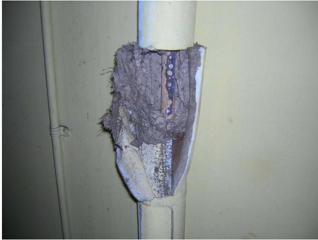
Figure 12.7 Asbestos pipe insulation showing multiple layers and penetration of wetting agent
