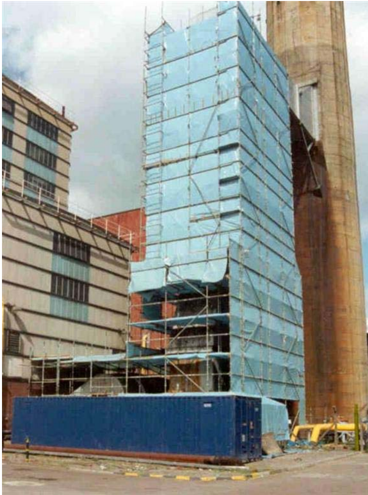
Figure 12.3 Enclosure for removal of lagging from a flue gas duct
