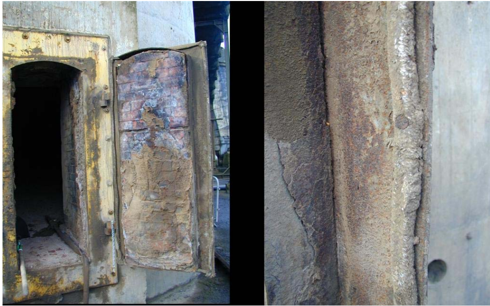
Figure 4.12 Asbestos rope sealing on chimney door. The image on the right is a close up view of the rope.
