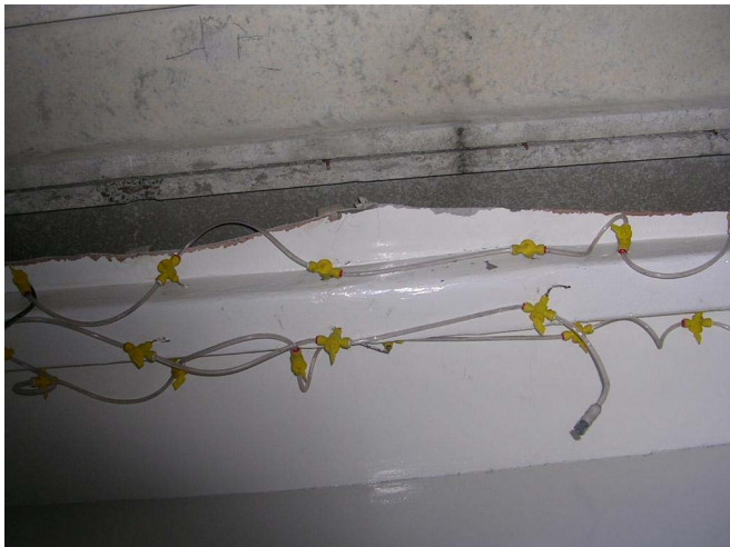
Figure 12.10 Example of multi-point injection used in wetting sprayed asbestos insulation.
