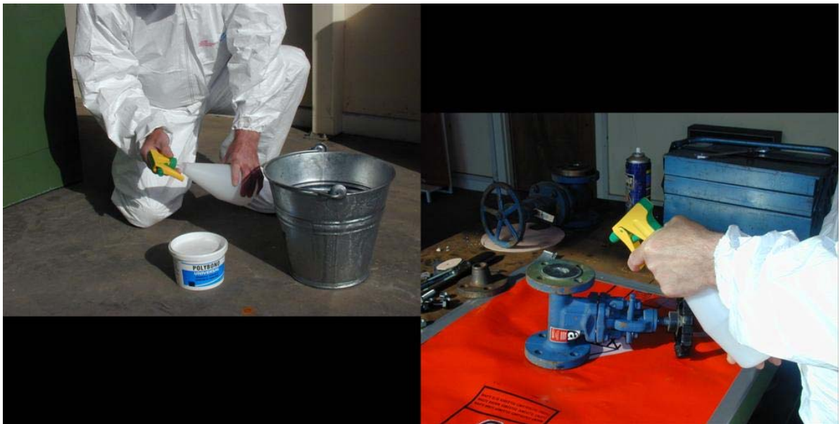
Figure 11.4 Dampening the asbestos gasket on a valve
